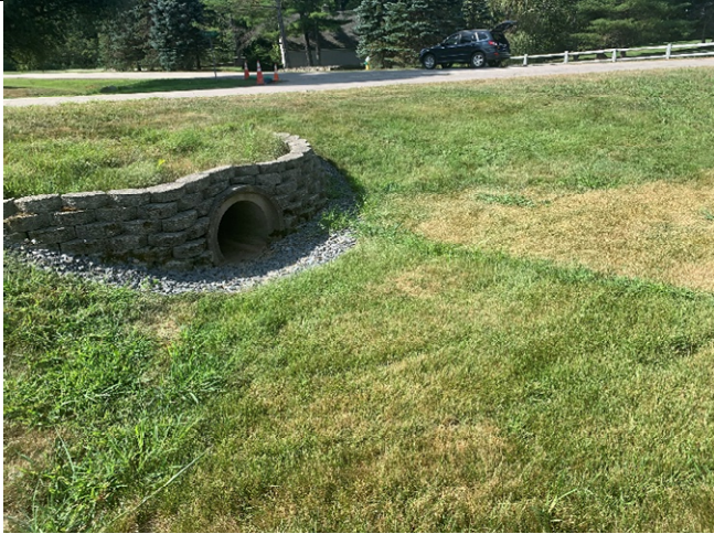
29 Gundalow -1 (Drainage Area)
