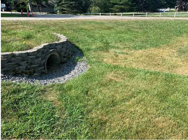
29 Gundalow - 1 (Drainage Area)
