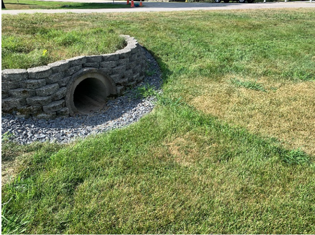
29 Gundalow - 1 (Drainage Area)
