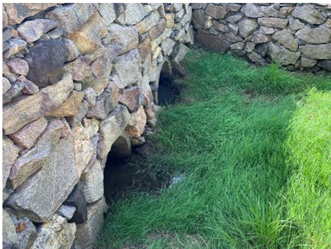
4 Brickyard Circle - 1 (Drainage Course)
