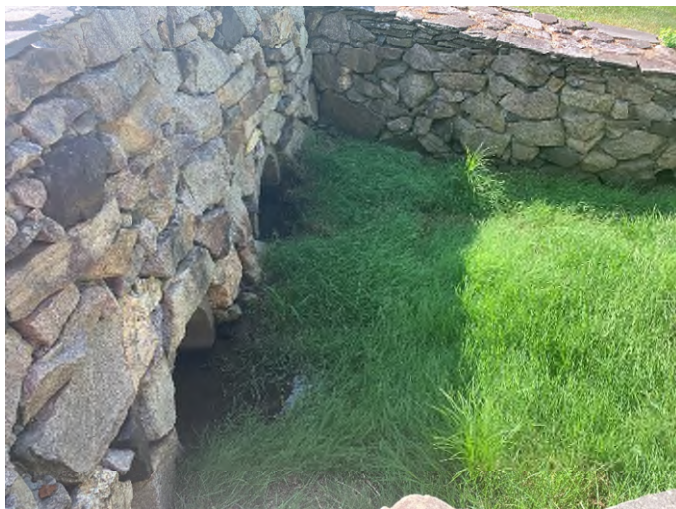
4 Brickyard Circle - 1 (Drainage Course)
